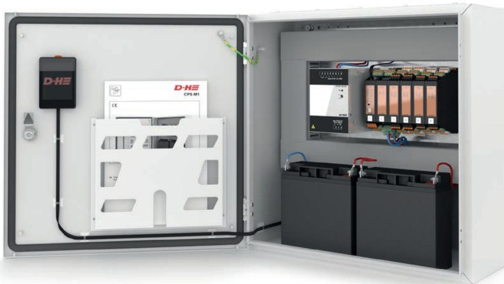
Fully modular and digital smoke vent control panel
